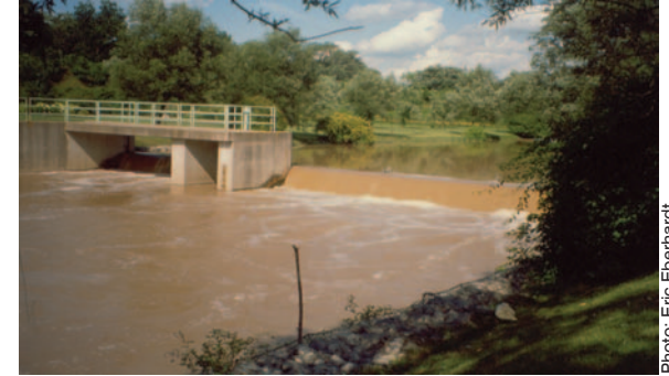
John Street Weir, Stratford
