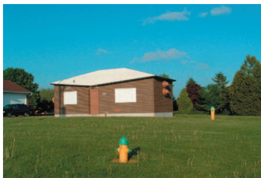
Mornington Street Well, Stratford
