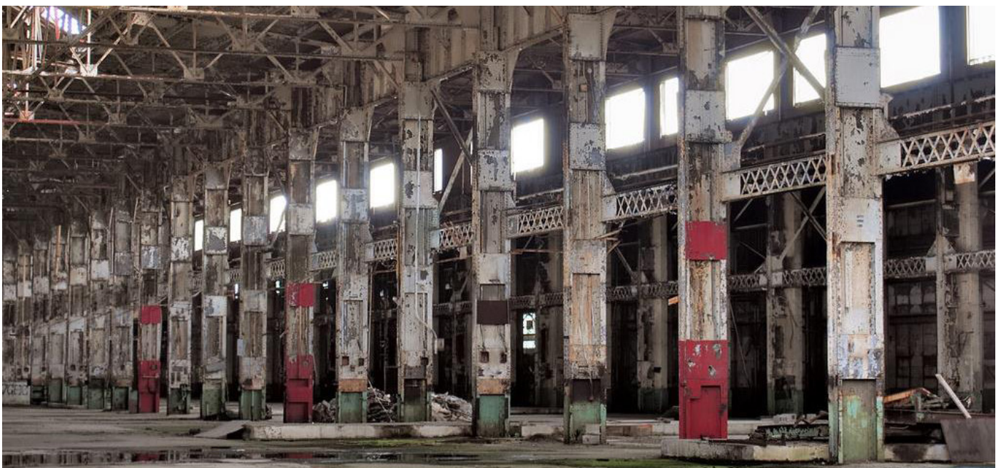
Figure 19 ► Grand Trunk Building interior
