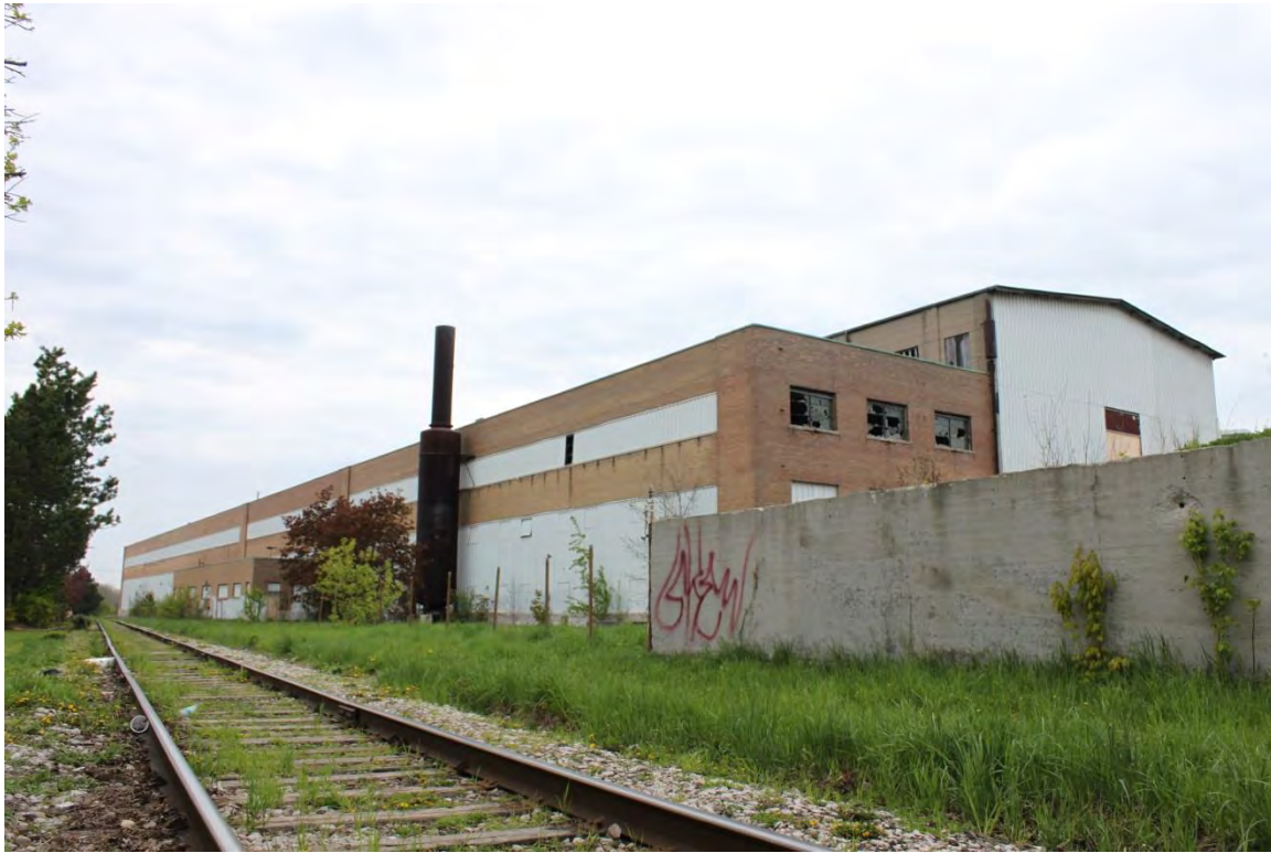
Figure A-5 View of exterior of building
