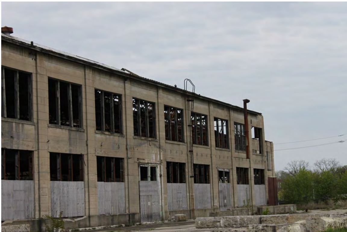
Figure A-6 Alternative view of exterior shell of building
