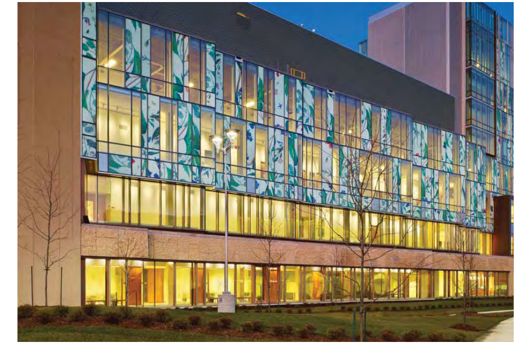
University of Waterloo School of Pharmacy - Waterloo, Ontario
