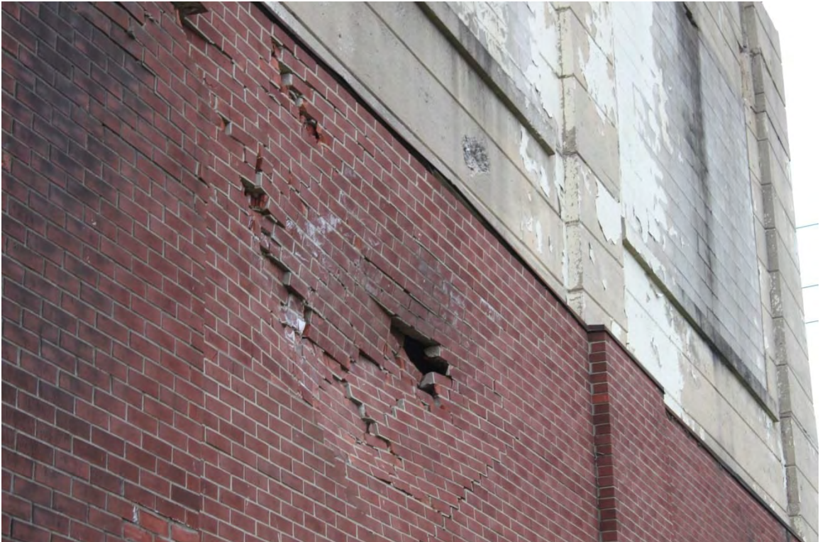
Figure A-6 View of building shell
