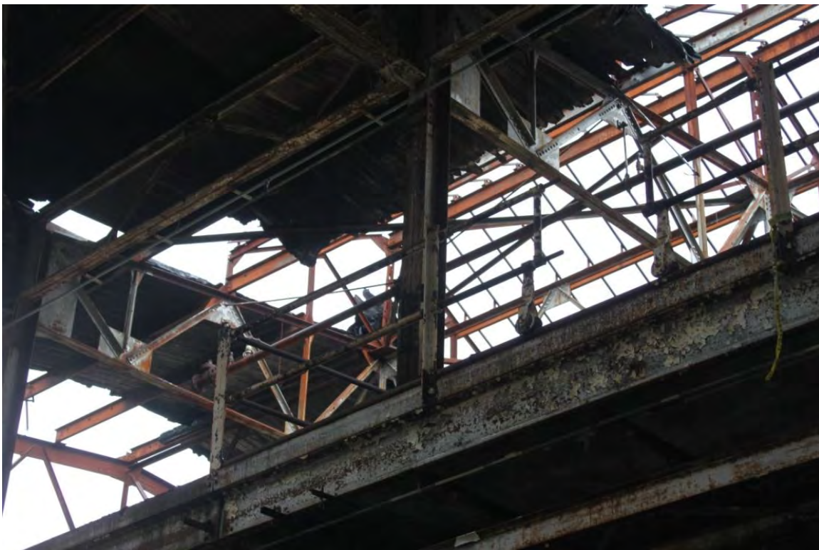
Figure A-13 View of an upper portion of the building shell
