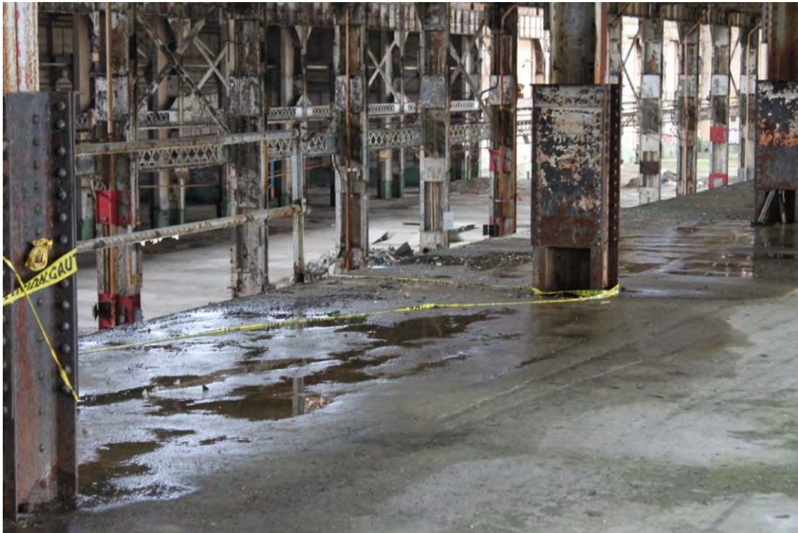
Figure A-10 View from the mezzanine
