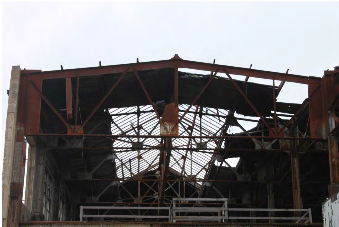
Figure A-7 View of roofing system and building structure
