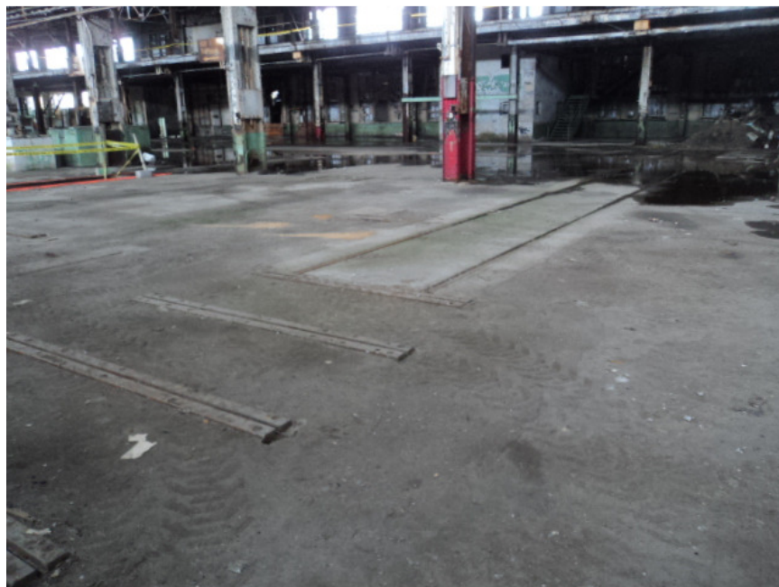
Photo #7: Typical embedded items in slab-on-grade
