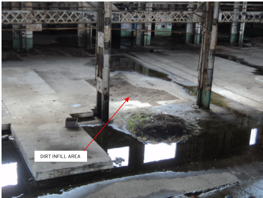
Photo #39: Typical slab-on-grade dirt infill area
