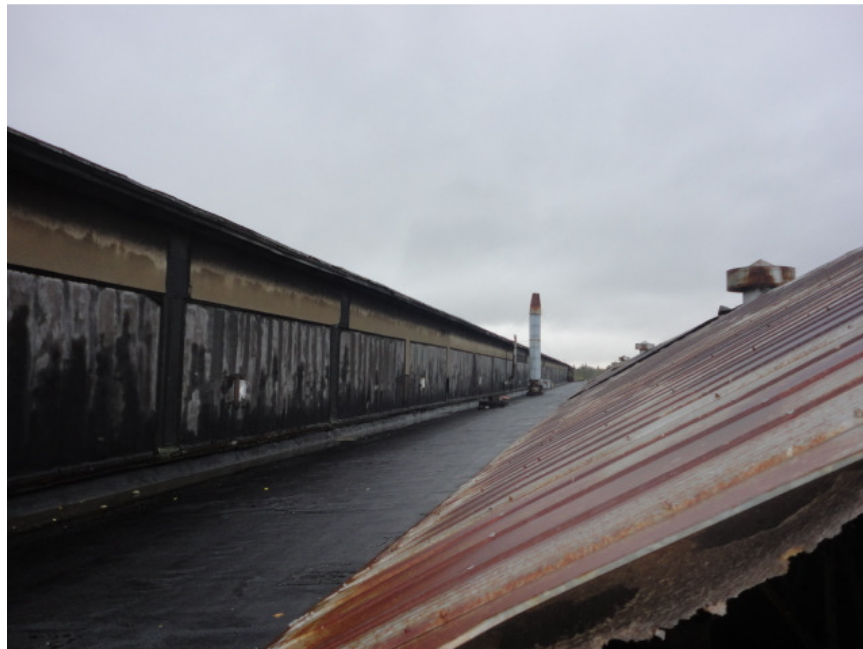
Photo #49: Typical roof assembly and condition
