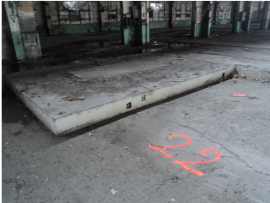
Photo #40: Typical slab-on-grade raised concrete pad
