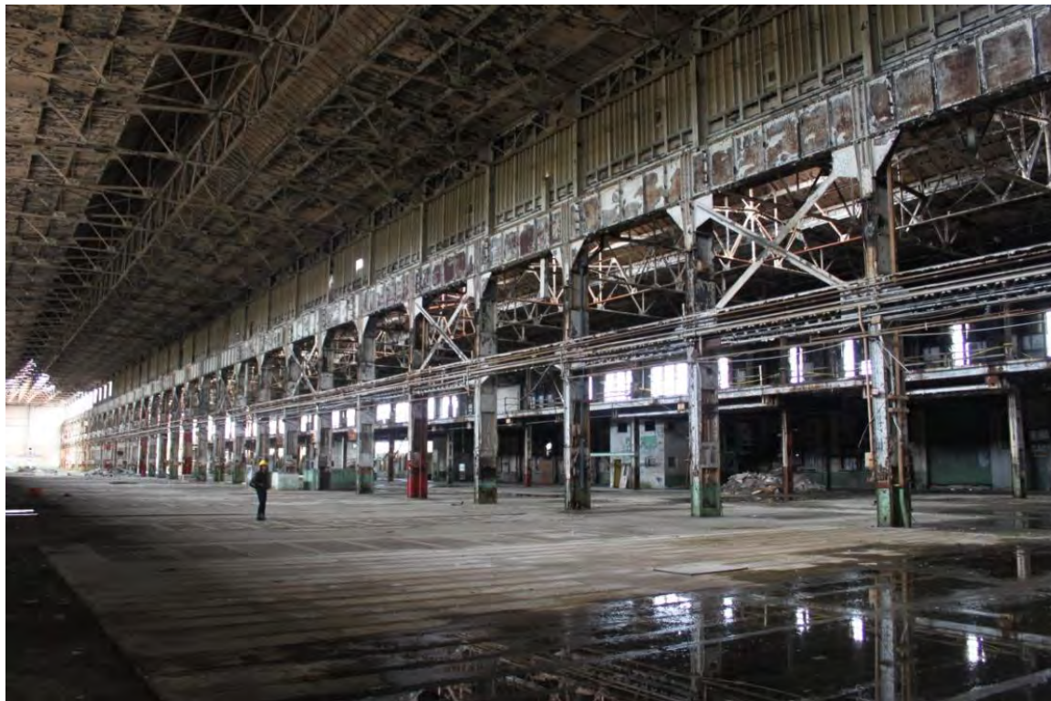
Figure A-8 Expansive view of the Machine Shop
