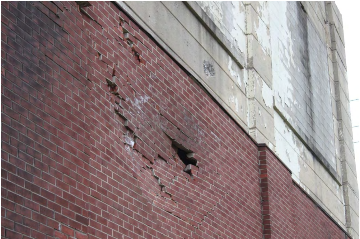
Figure A-6 View of building shell
