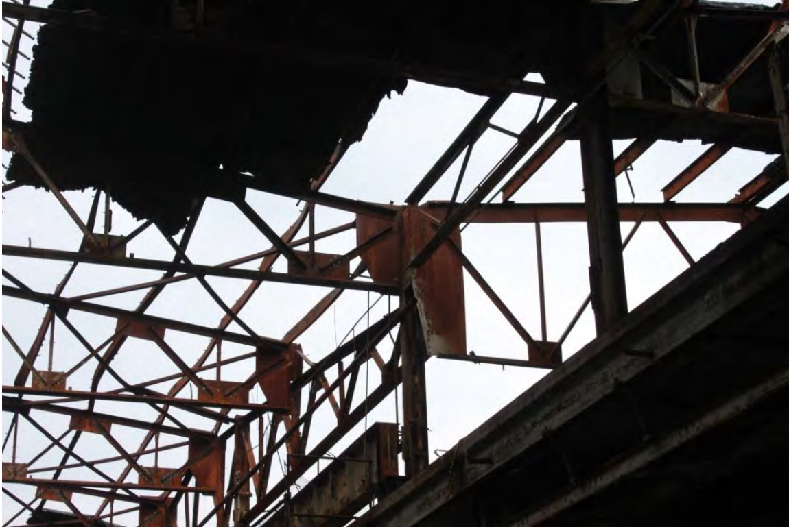
Figure A-12 Alternate view of roofing system and building structure
