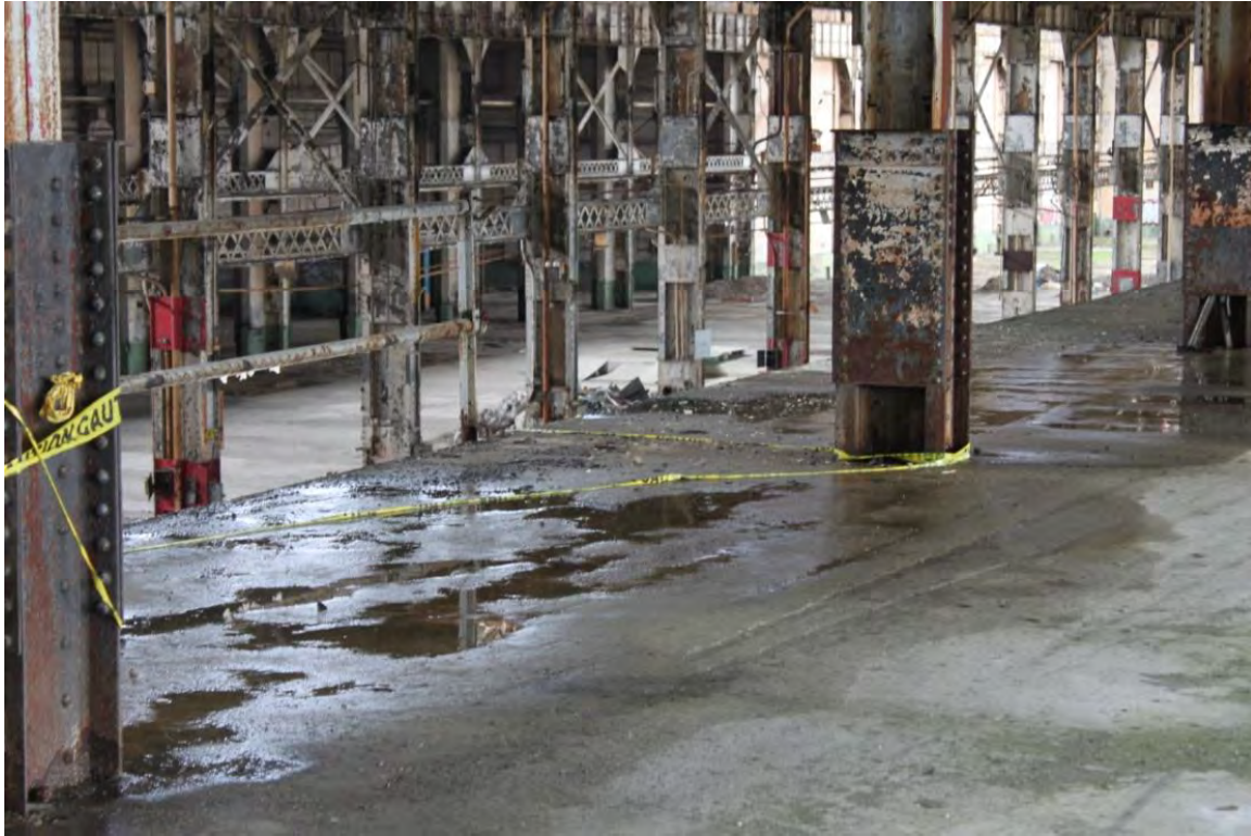
Figure A-10 View from the mezzanine
