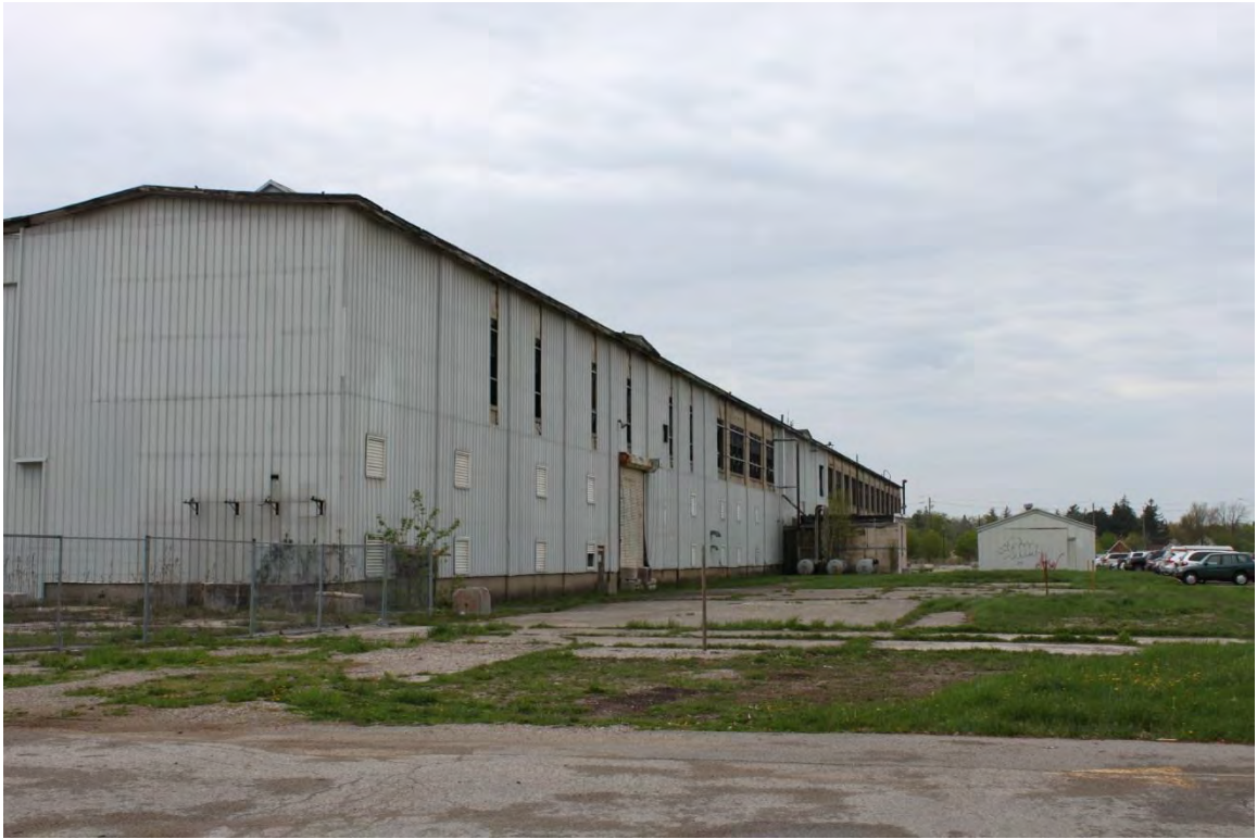
Figure A-5 View of portion of structure of site
