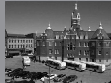
Typical day-to-day conditions
