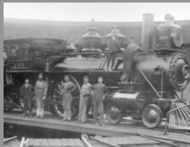
Stratford's railway heritage
