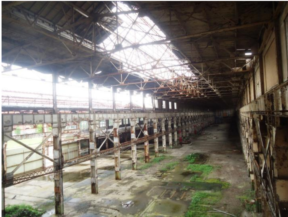
Photo #1: General Overview of the Structure
